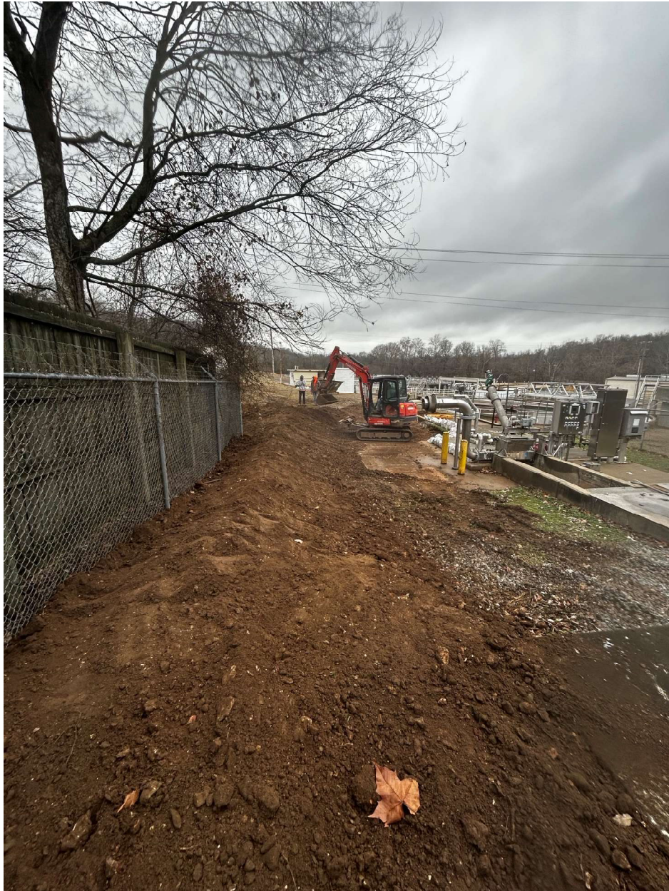
Berm construction limiting offsite stormwater flow (2)
