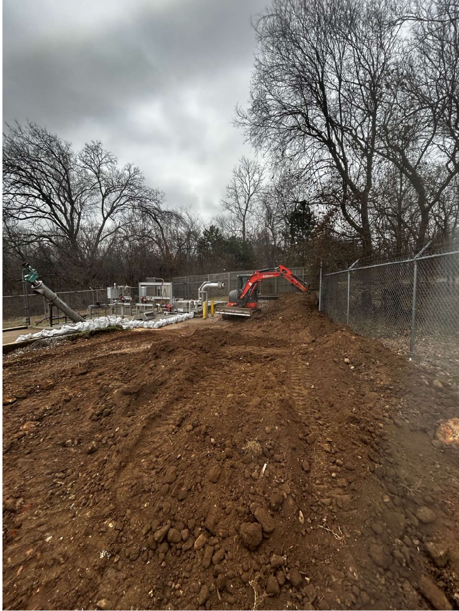
Berm construction limiting offsite stormwater flow (1)
