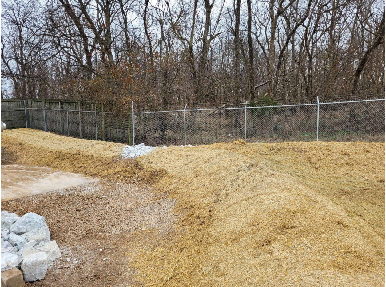
Completed berm construction on February 10 th , 2025 (1)
